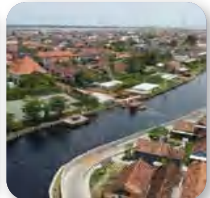
Proyek Pengadaan dan Pemancangan Loji Banger Jawa Tengah Procurement and Piling Project of Banger Loji Central Java
