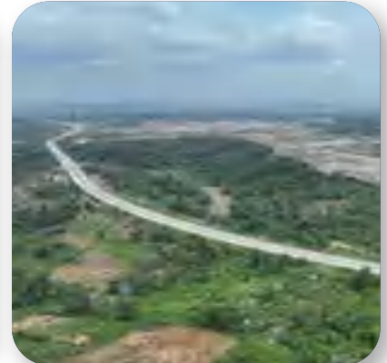
Jalan Tol Jakarta Cikampek II Selatan Seksi 2 DKI Jakarta, Jawa Barat Jakarta South Cikampek II Toll Road Section 2 DKI Jakarta, West Java
